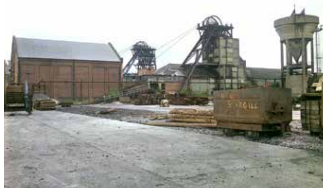
Betteshanger Colliery after closure. Photo Nick Catford
